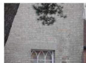
White brick: Flemish bond
